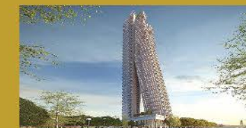
Altair, Colombo An iconic landmark of 13 lakh sq ft, designed by internationally celebrated architect Moshe Safadie.
